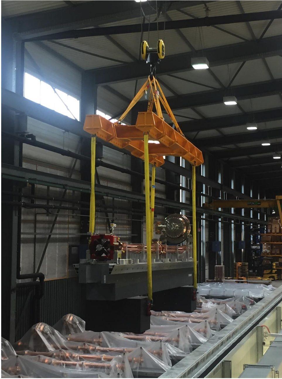
Movement of girder into assembly hutch
