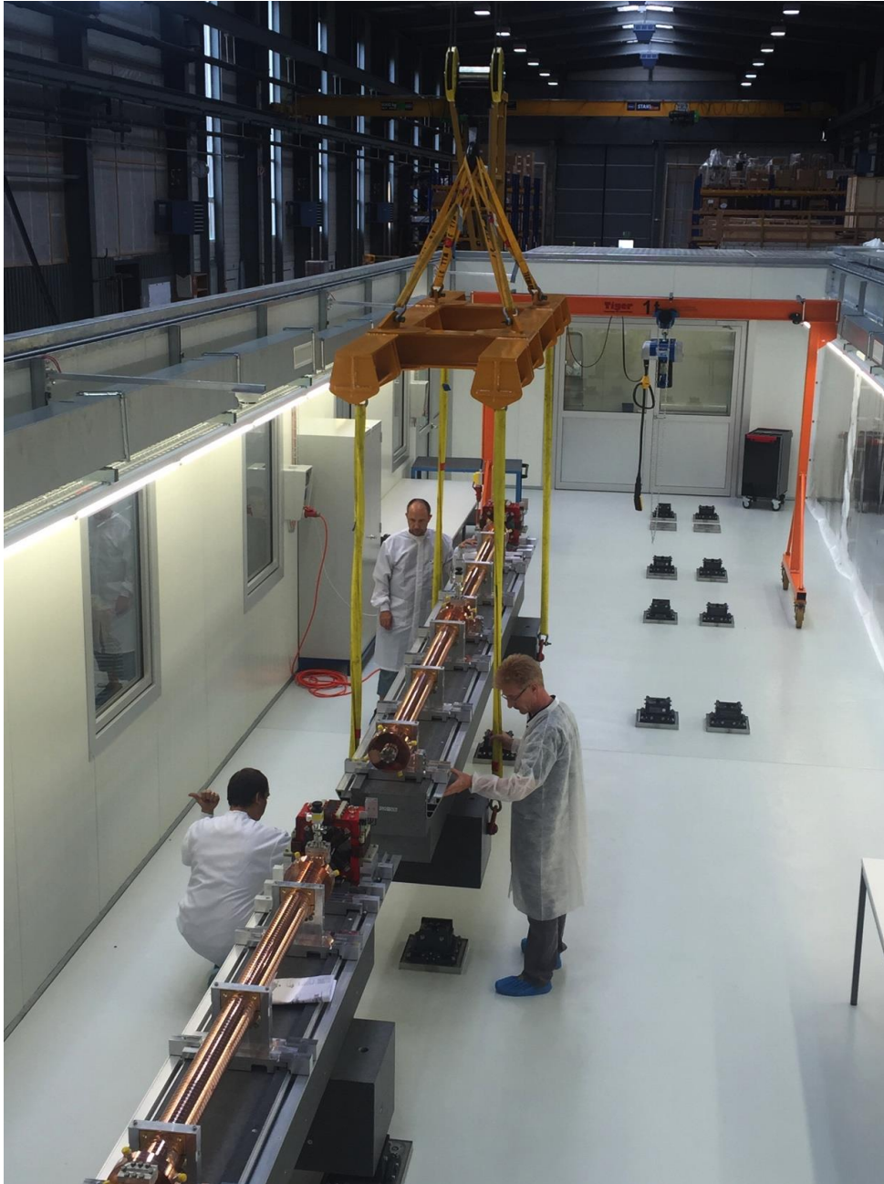
Installation of girders into assembly hutch
