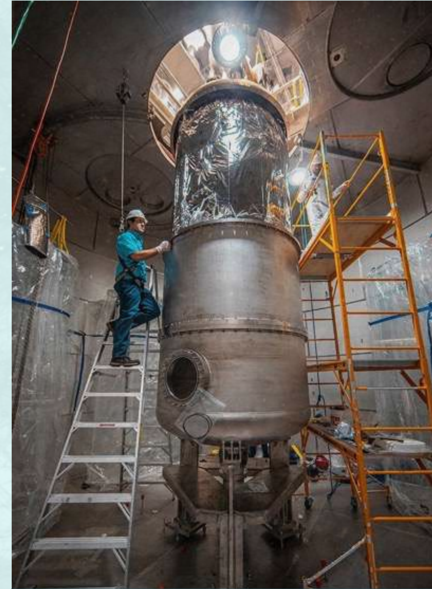
ICV installation in OCV
