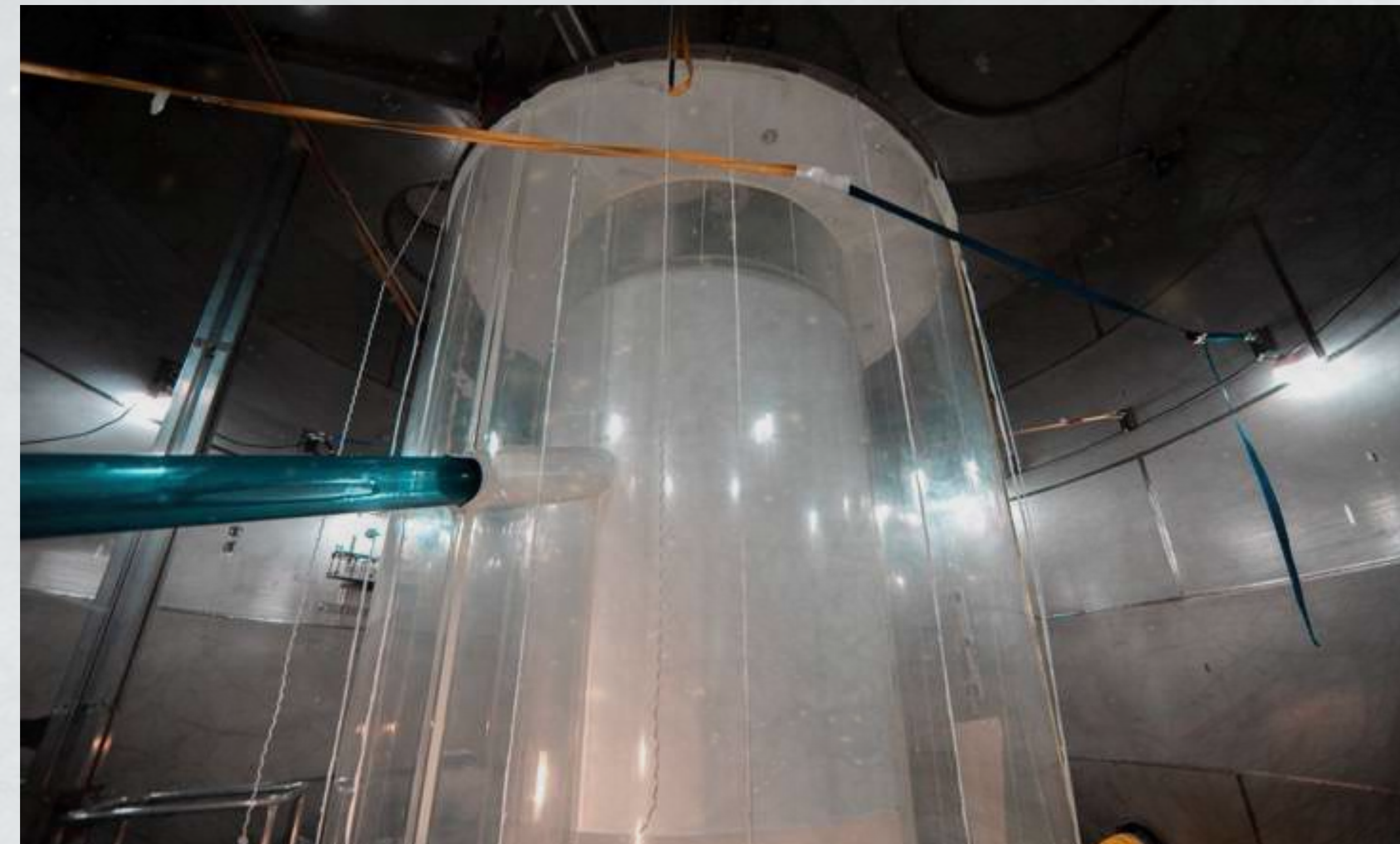
Installation of OD tanks around Outer Cryostat Vessel
