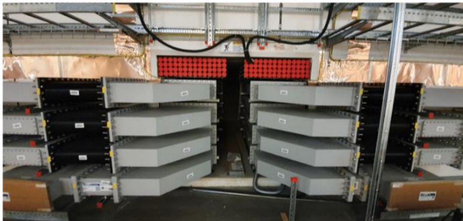
SCL RFDS, Tunnel
