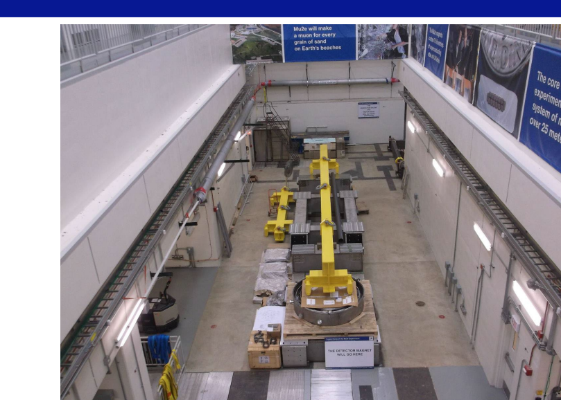
Mu2e experimental site in construction @ Fermilab
