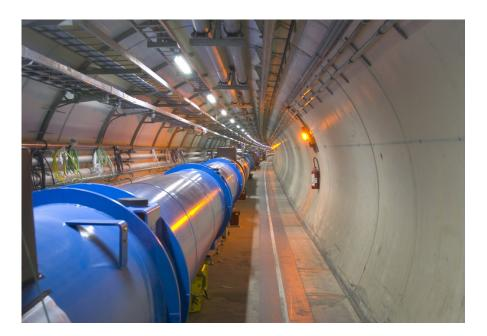
To reach the required energy in the existing 27 km tunnel, the super conducting magnets operate at **83 Kilogauss** (200'000 x Earth's field) in super fluid helium.
