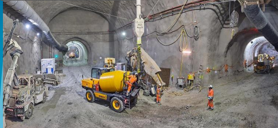
US/UW57 cavern with entrance to UR55 and UA57 galleries
