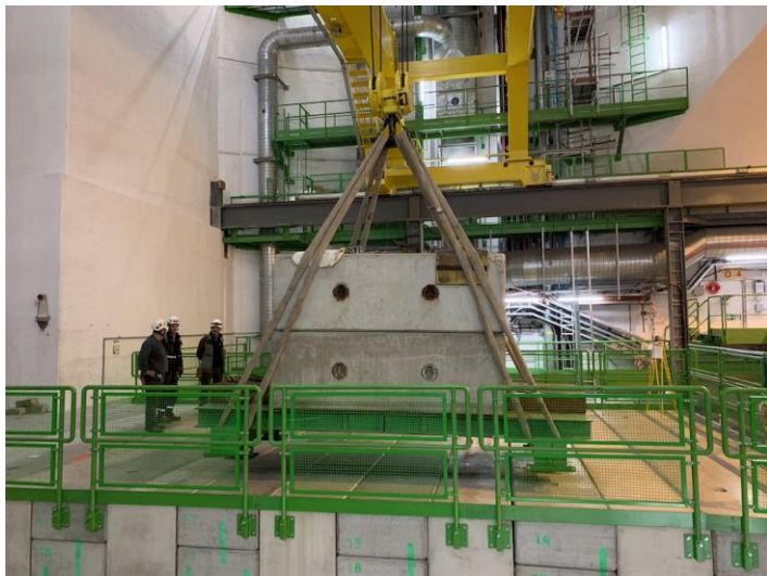
Load test UX25 crane
