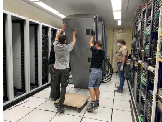
Removal old racks
