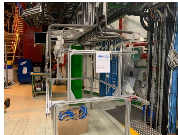
ITS cooling pipes and plant mockup
