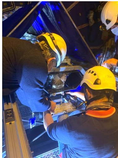
Install micrometric adjusting tables (Tue-Wed)
