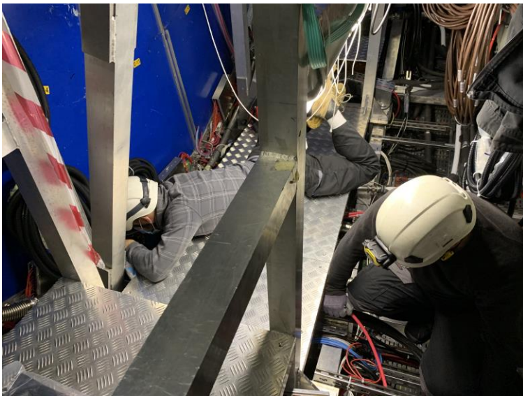
Cooling, LV, HV, Ethernet connected
