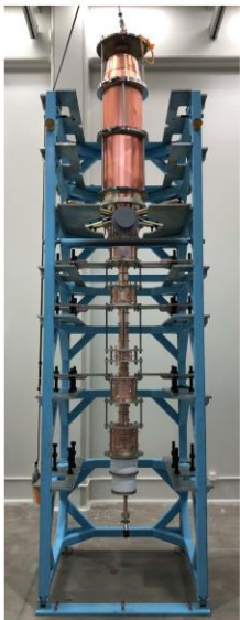
Klystron welding completed on Oct. 20, 2019
