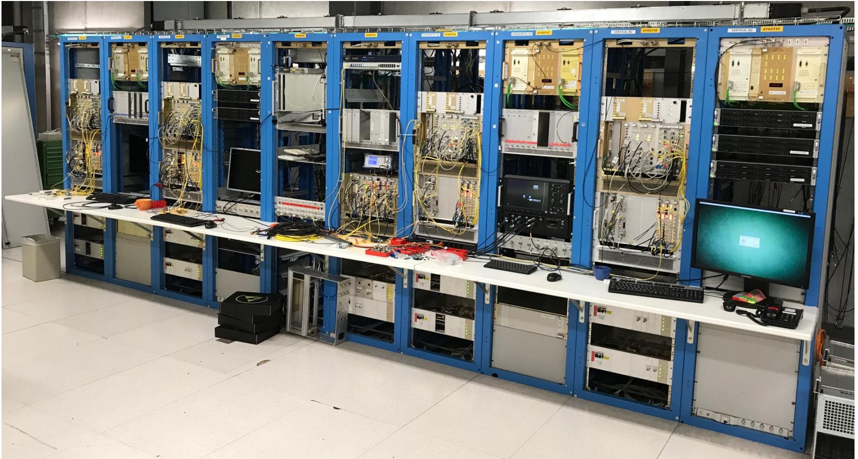
Pre-LS2 ADT Low Level RF system installed in LHC point 4. Beam position measurement, digital signal processing, all ADTObsBoxes.
