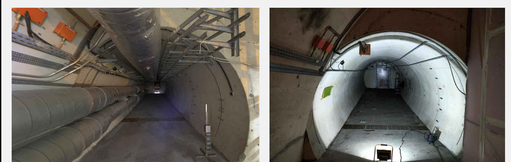
T112 before and after removal of pipes.
