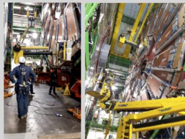
4: Hoist with crane
