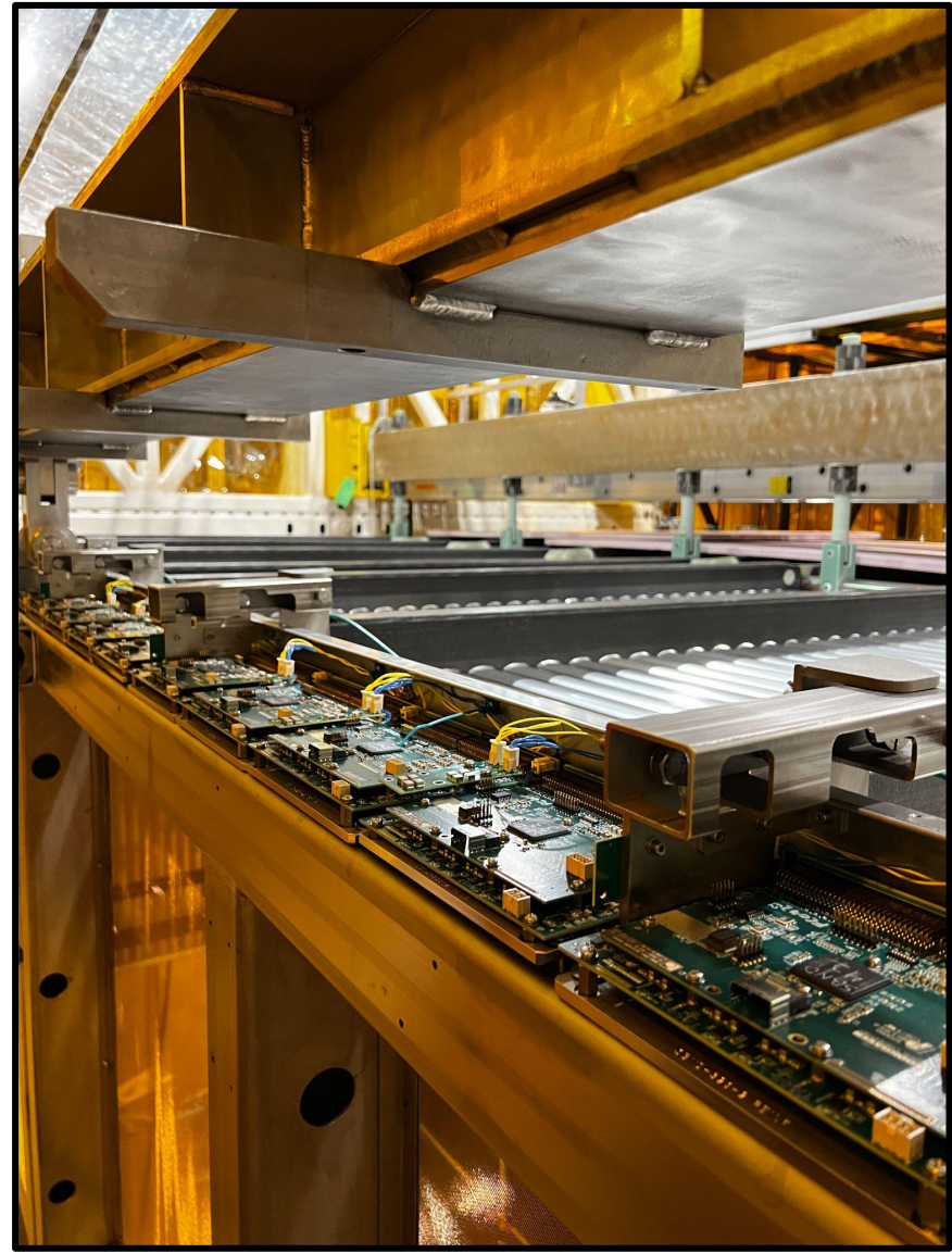
Installation of Cold Electronics, December 2021 & May 2022
