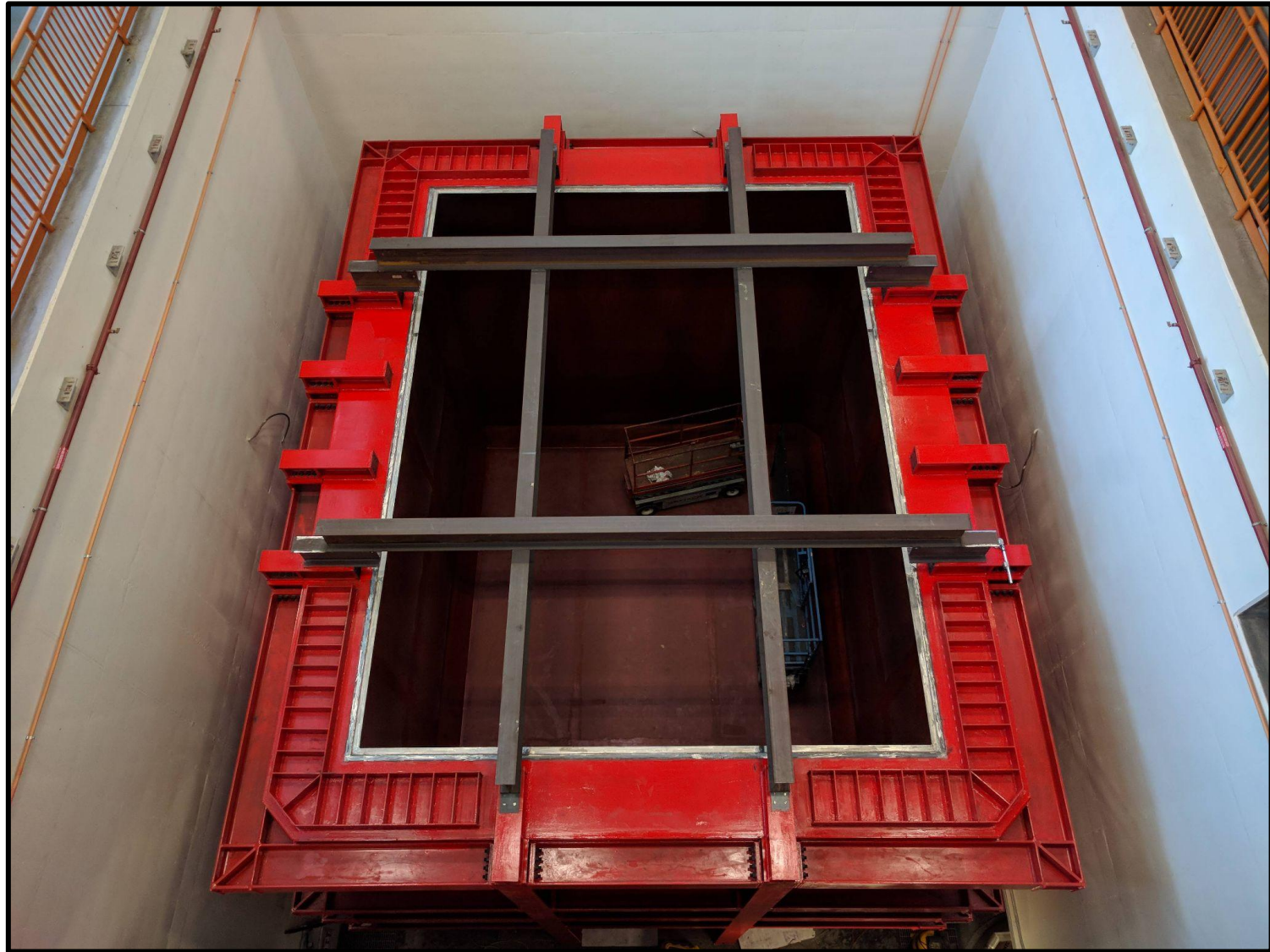
Cryostat outer shell completed, November 2019
