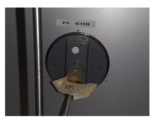
Leak on the PI 6119 is 115 ppm
