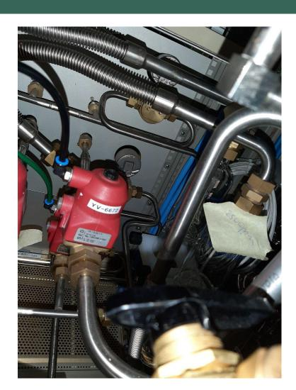
Leak through the valve YV6672 is 2500ppm
