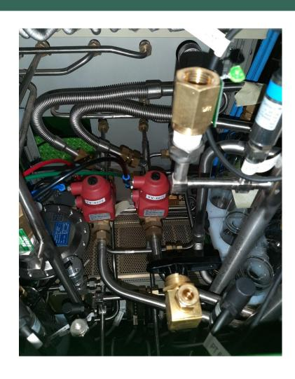
Leak on the valve YV 6272 is 150ppm and on the YV 6271 is 180ppm
