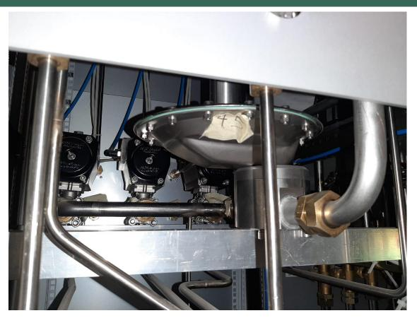
Leak on the head of the Zimmerli in the lower side of the rack is about 45 ppm
