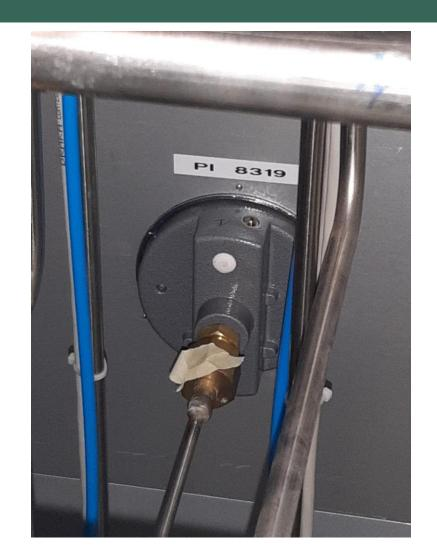
A leak on the connector of the PI 8319 is 40 ppm
