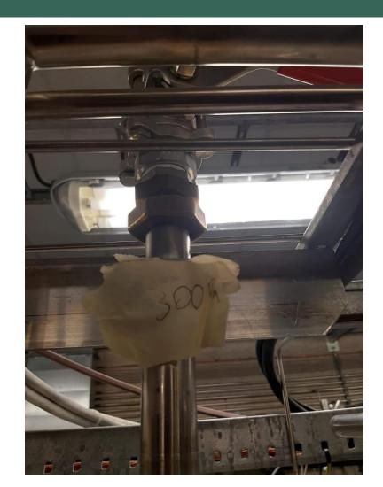
Leak on the valve above the RPC Purifier 3 rack in the SG is about 300ppm
