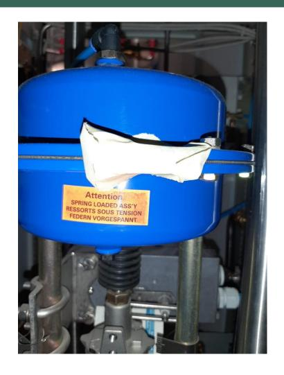
A leak has been found on the head of the Von Rhor Valve inside the pump Rack but is not present anymore
