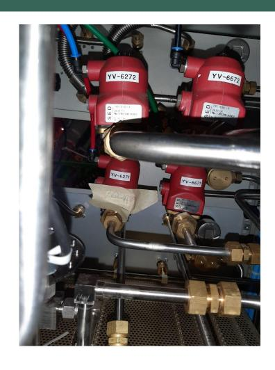
Leak on the valve YV 6271 is 200ppm
