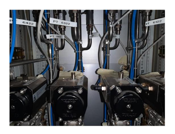
Leak on all the pneumatic valve's connectors directed to the front panel, from left to right the leaks are 102 ppm, 910 ppm, 1393ppm, 910 ppm.
