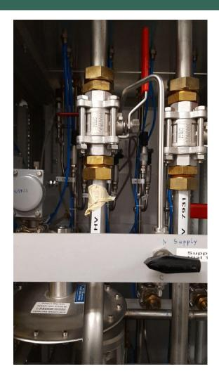
A leak on the connector of the HV 8331 is 49 ppm
