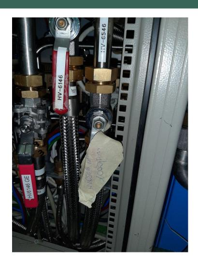
Leak on the valve HV 6546 is 1000ppm
