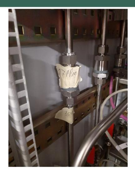
Leak on the no-return valve in the RPC mixer the leak on the upper connector has benne closed and the leak on bottom connector is 400 ppm
