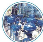
CRYOGENICS 2 new large 1.9 K helium refrigerators for HL-LHC near ATLAS and CMS will allow cryo-separation between arcs and triplet regions.
