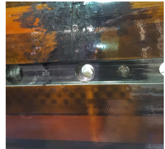
Result of electrical short circuit quench heater to coil in a Nb 3 Sn coil
