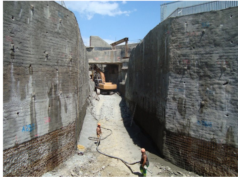
Transfer line under TP9
