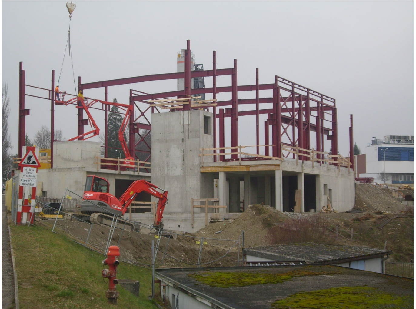
Start construction equipment building (klystron hall)
