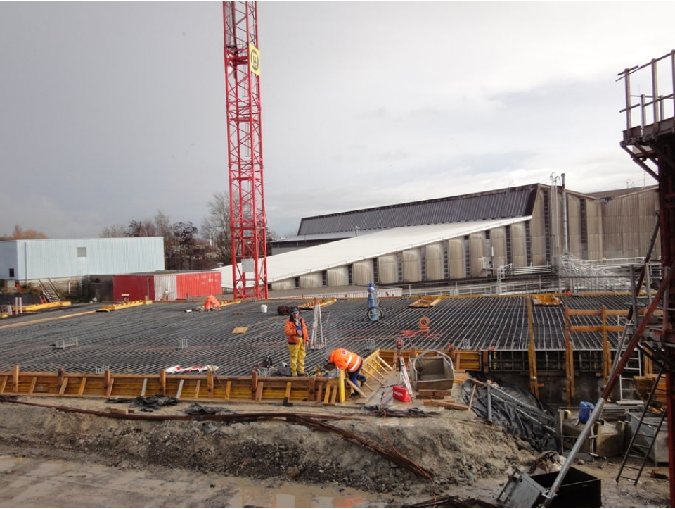
Klystrons building slab
