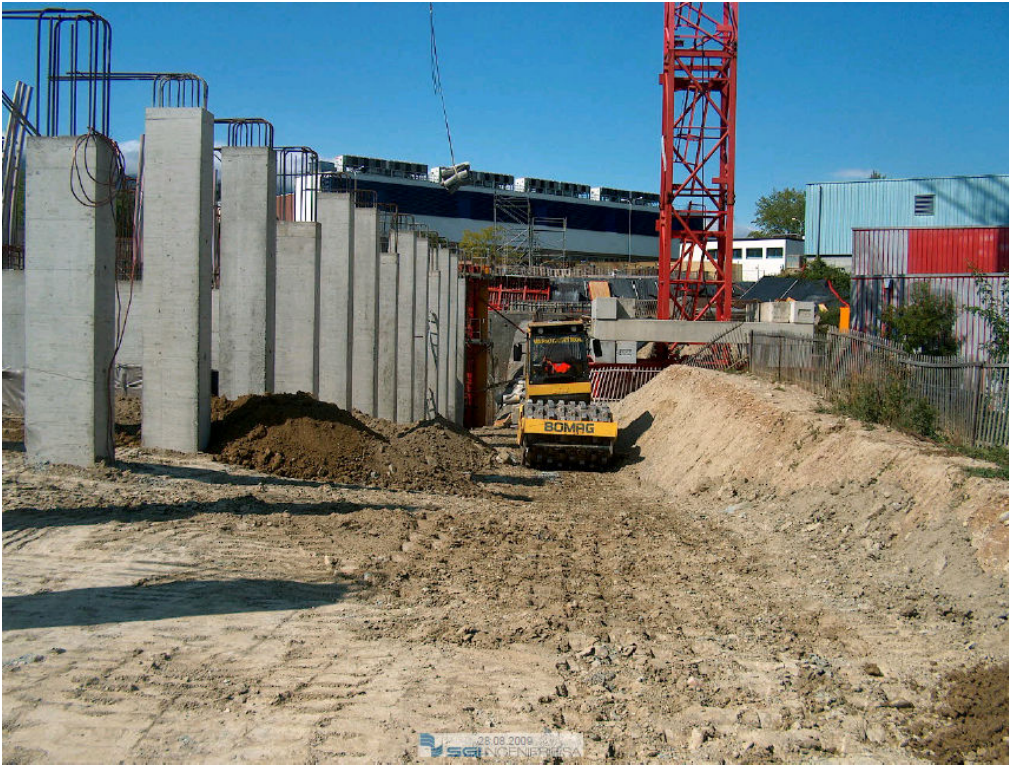
Concrete works of wave guides and backfilling
