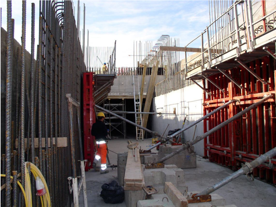
Concrete works of Linac 4 tunnel
