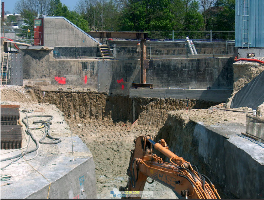
Low energy structure concrete works
