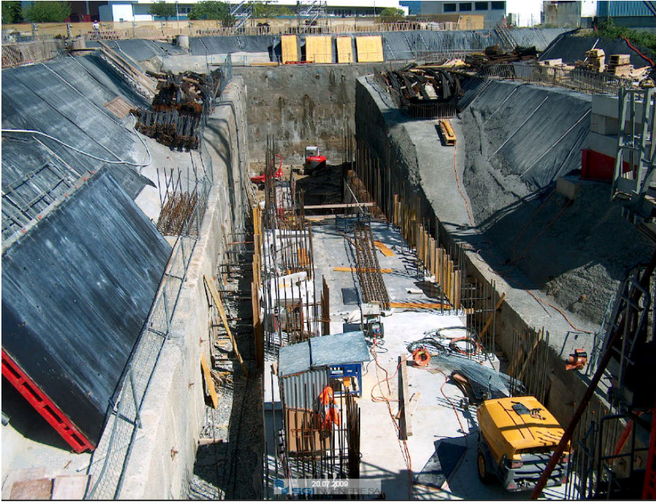
Concrete works of Linac 4 tunnel
