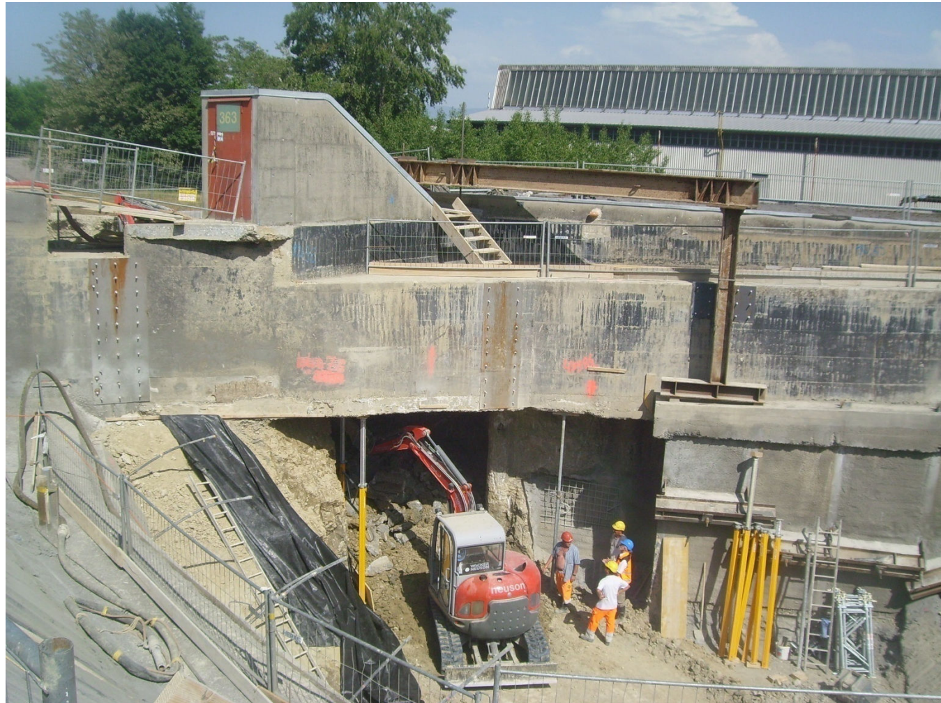
Transfer line under TP9
