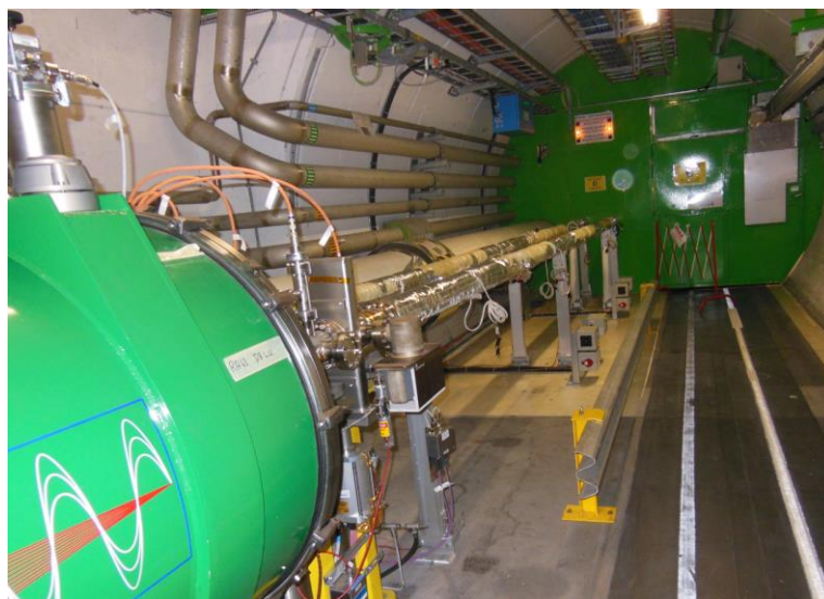
Figure 9: - Vacuum sector B5L4 during YETS 2017/18
