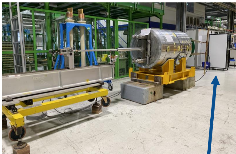
Connect all cable needed to the electronic rack
