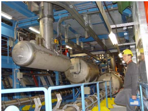
Proximity cryogenics equipment for the magnets and the liquid argon calorimeters
