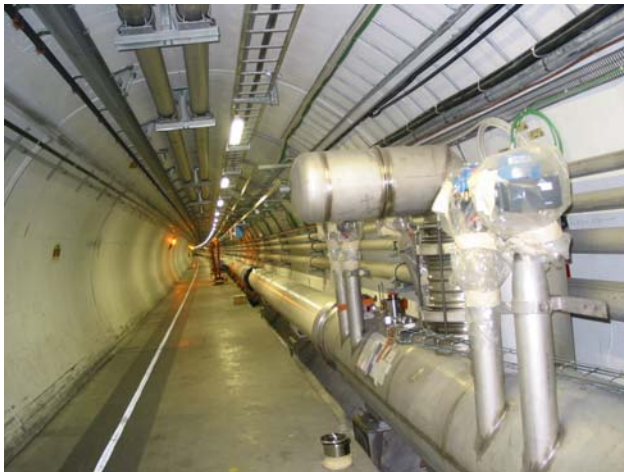
QRL (no magnets attached yet)
