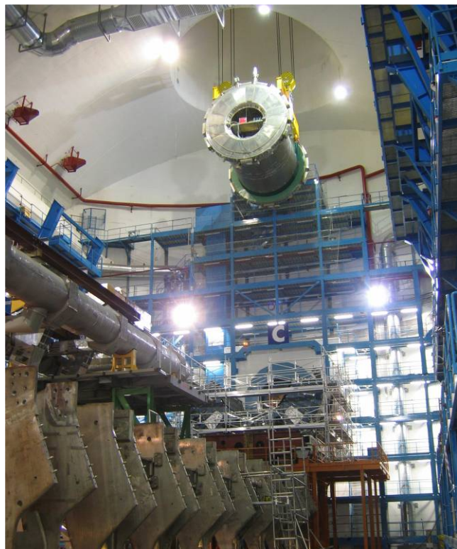
Nov. 2004: Barrel lowering in ATLAS pit
