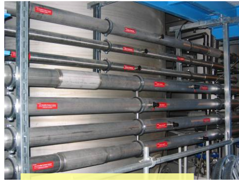
1.3 km interconnecting LAr & LN 2 transfer-lines
