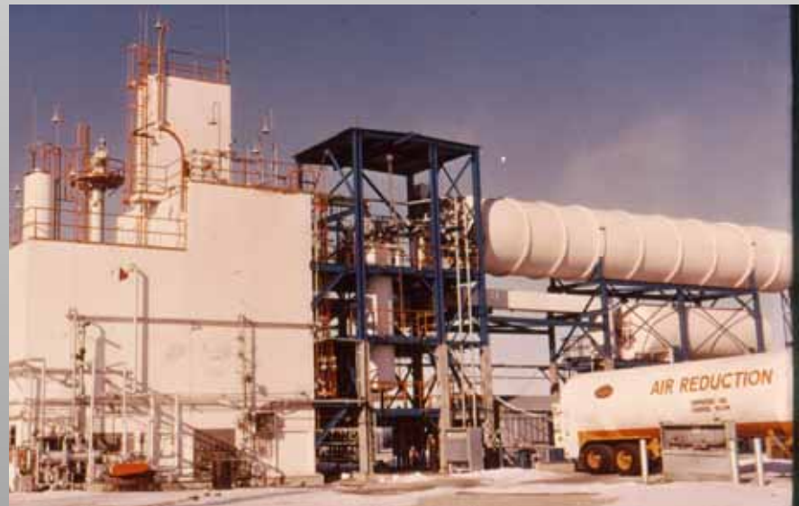
800 l/h helium liquefier in Otis, Kansas, built in 1966
