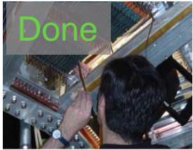
Remove Services and FEE (outside cleanroom)
