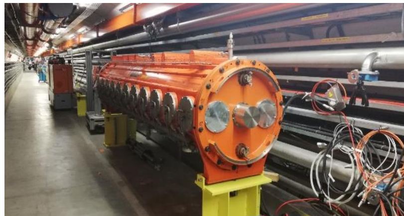
Re-installation of magnets and RF cavities in LSS3
