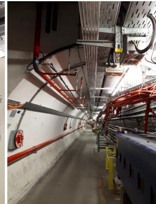
WP2, 3 & 4 installed in LSS5
