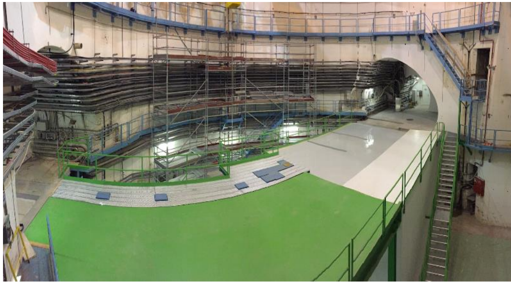
CE works in ECX5 complete on time.
