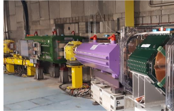
New extraction line bending magnets
