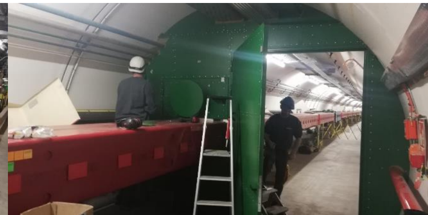
WP1 installed in LSS6+
