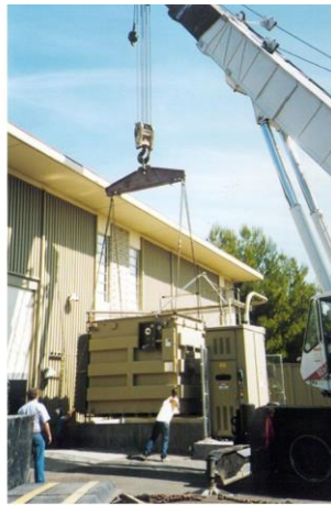
PEP-II 1.2 MW klystron and HVPS
