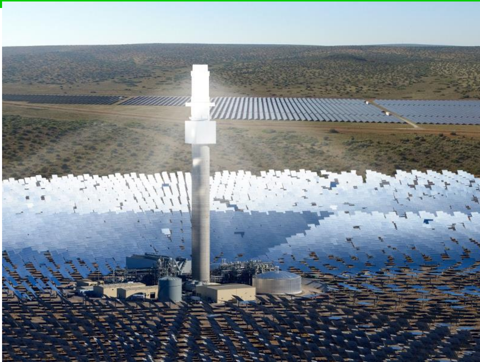
CSP Plant in South Africa
