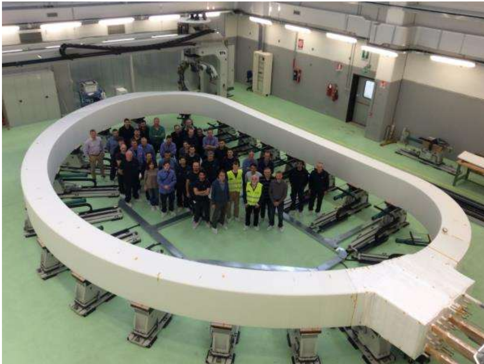
First TF winding-pack before resin impregnation
