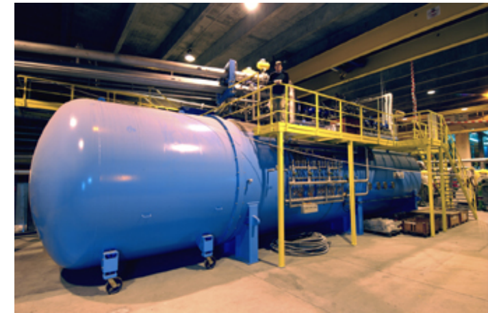
Coldbox of the 4.5 LHC refrigerator
