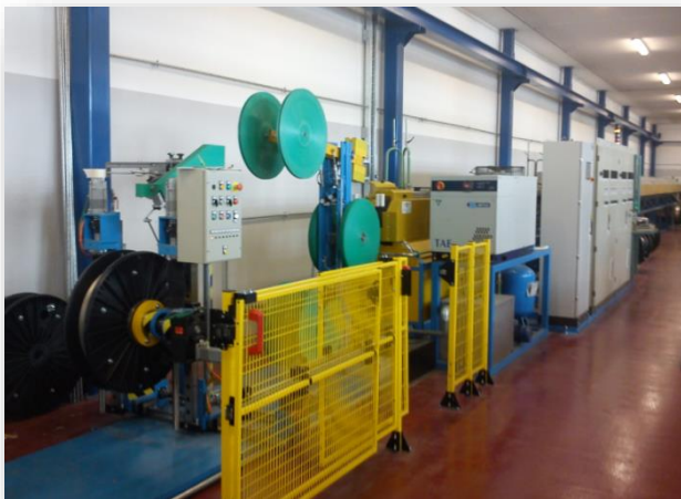
20 m long in-line furnace
