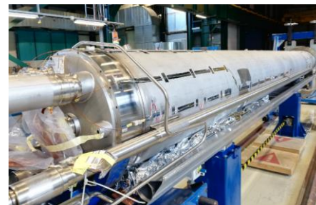
Installation of PT100 on outside surface of CM shells
