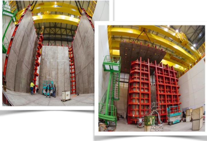
Construction of the outer structure
