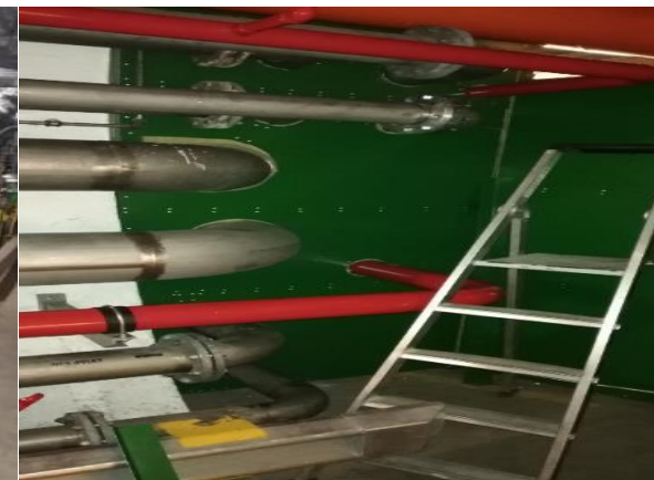
Fire Safety doors being finalised
