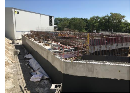
SF57: Wall casting
