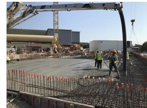
SHM57: Ground slab casting
