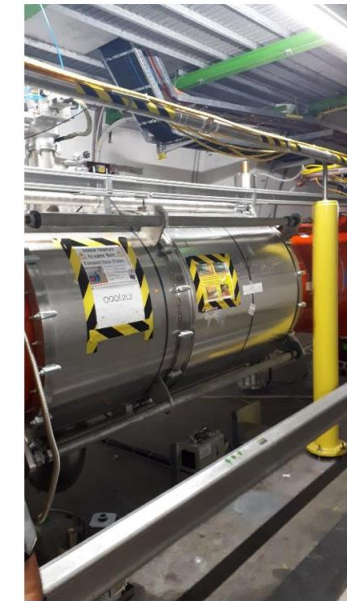
Tied-rod installation at IT2
