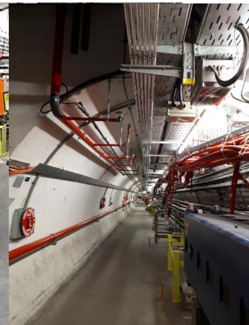
Fire Safety being completed
