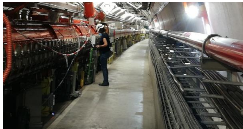
Magnets and RF cavities in LSS3 installed, commissioning to start shortly
