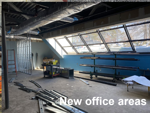
New ductwork
