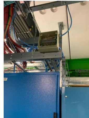
Junction box for accidentally cut P-sensor cable
