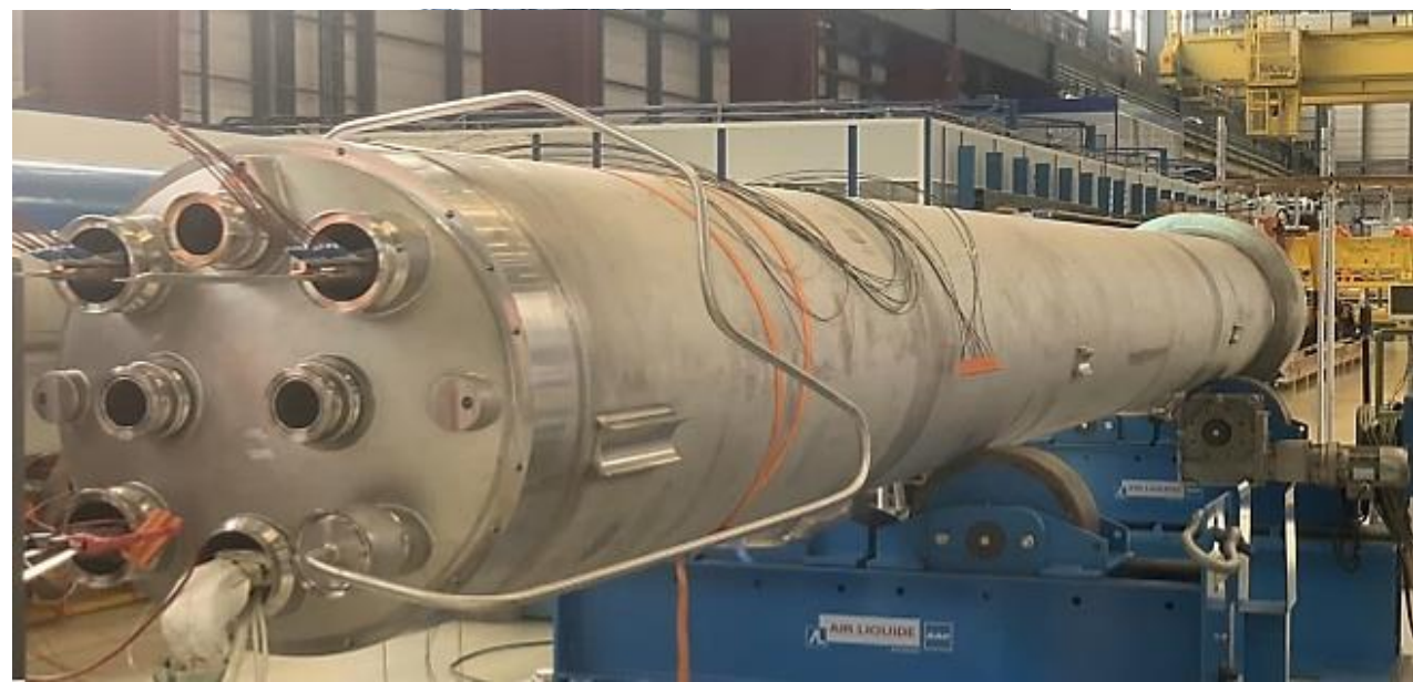
S5 in construction in LMF
