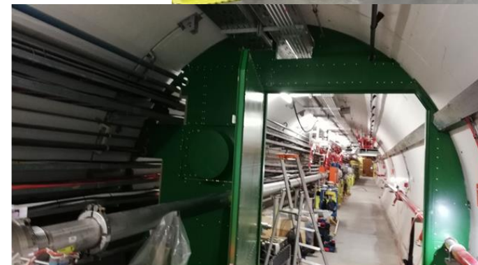
WP1: Final fire door installed in LSS5
