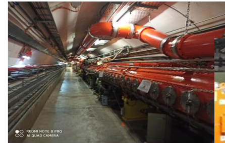
The new RF cavities in LSS3
