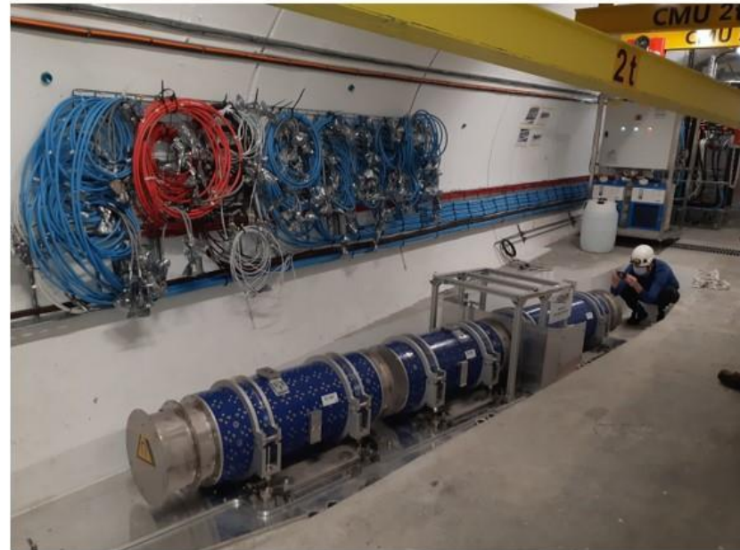
Pictured: the three magnets installed in TI12 (LHC)
