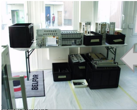
Cleaned components waiting for reinstallation in gallery
