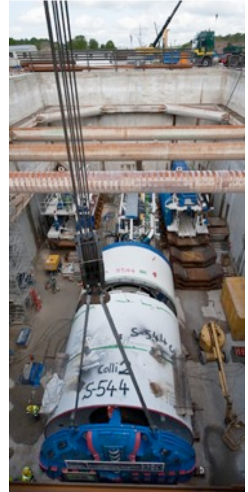
Lowering into hall
