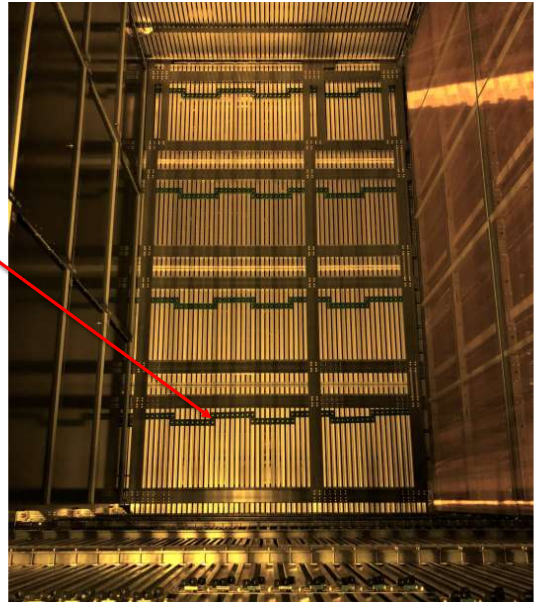
Upstream End Wall next to TCO
