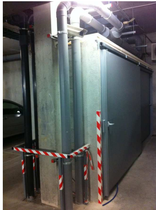
Passage of the piping through the ceiling
