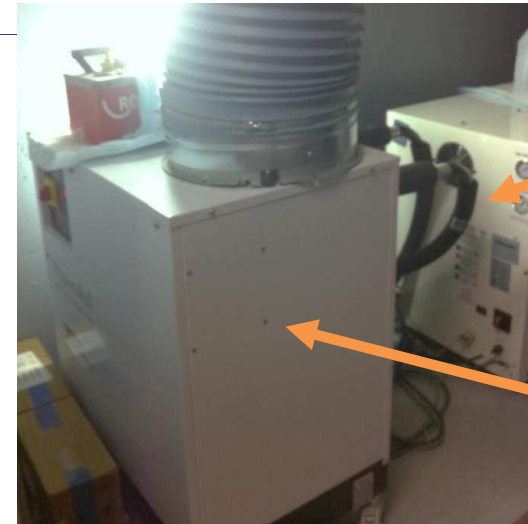
Chiller (water temperature at 18°C)
