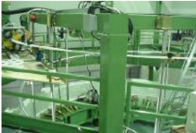
Conductor spiral leading into cylinder
