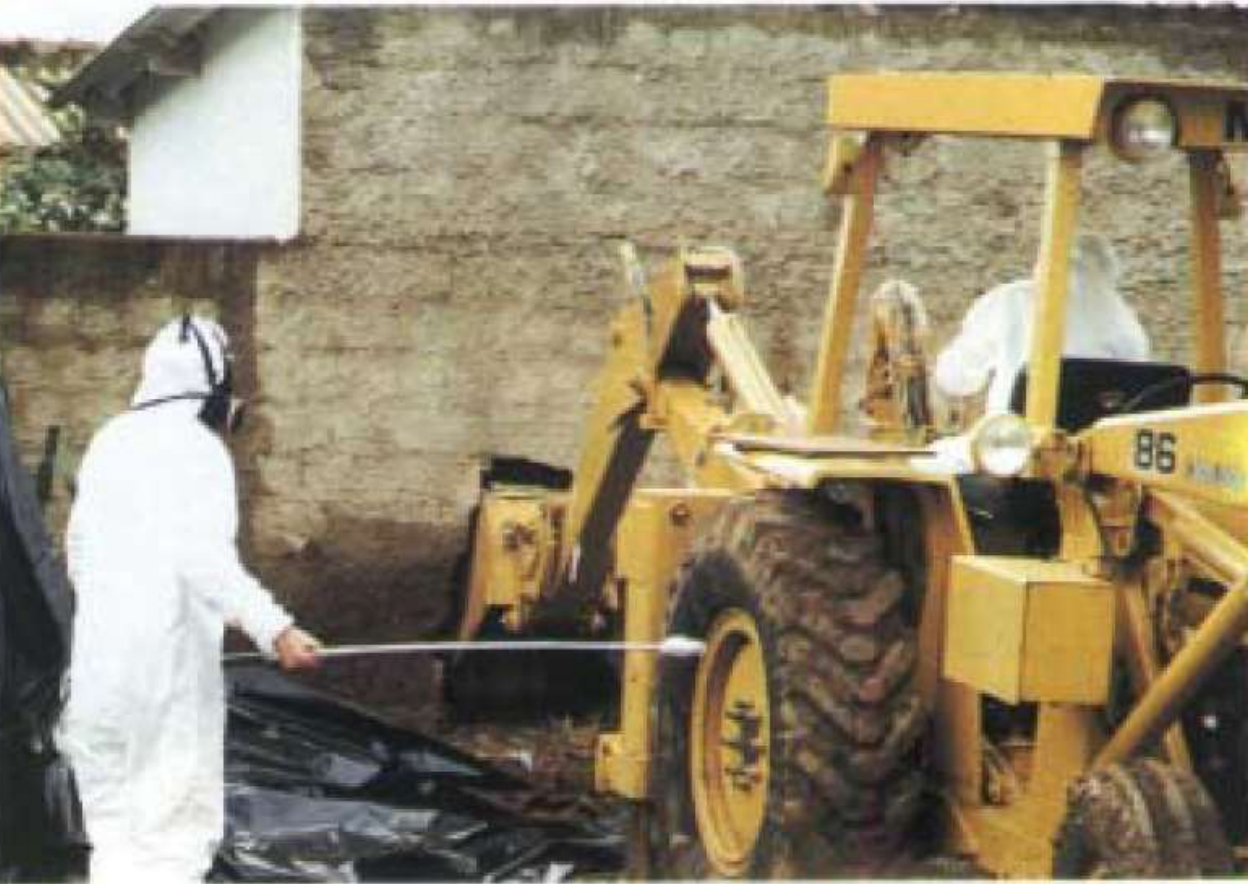
10. A hole is made to remove a radiation hot spot giving a dose rate of 0.5 \text{ Sv}\cdot\text{h}^{-1} .
