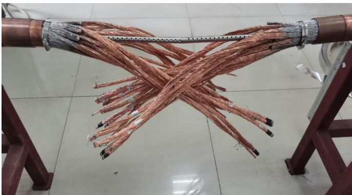
Central cooling pipe installation
