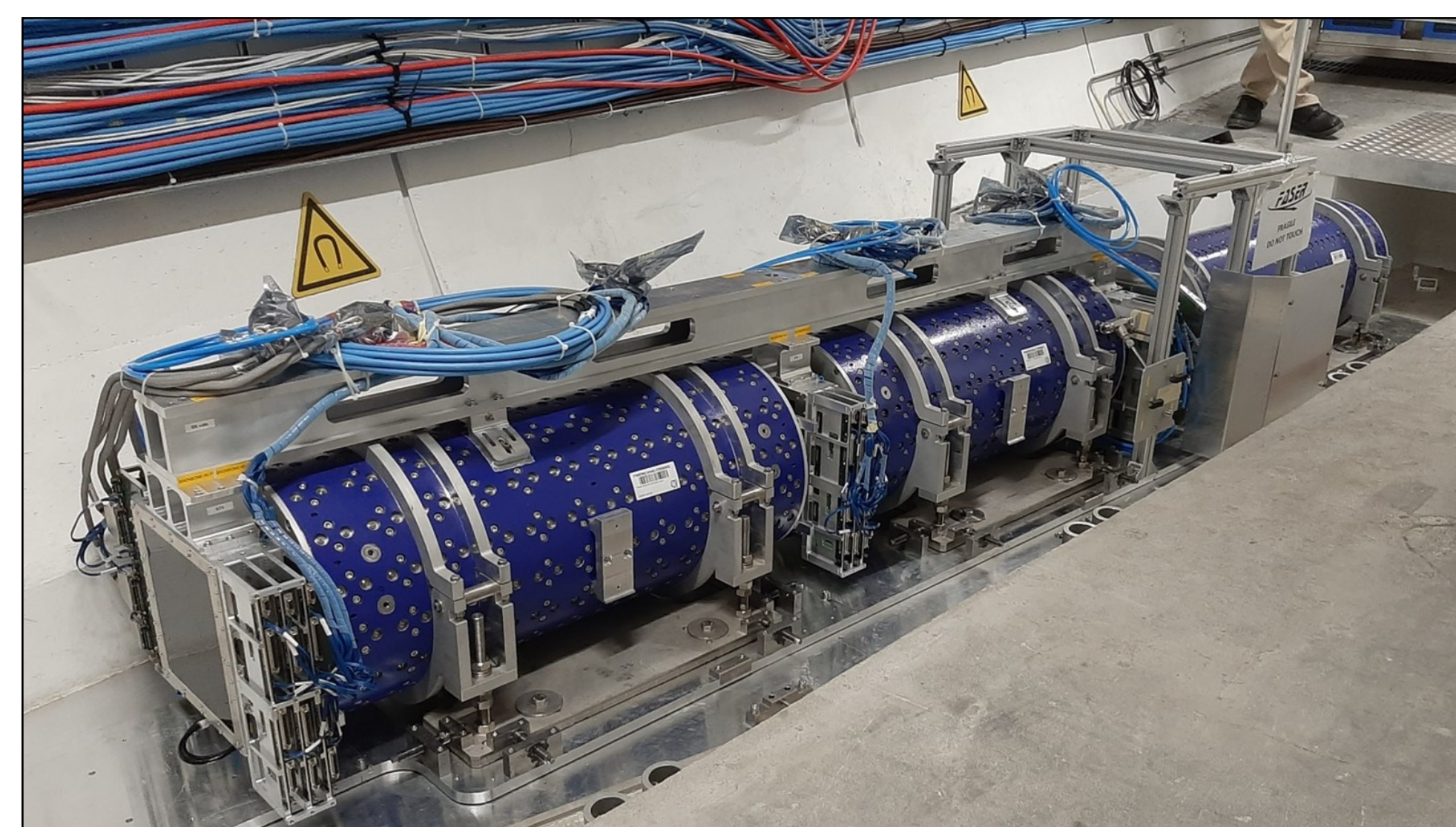
Fig. 2– FASER permanent magnet dipoles installed in LHC, 480 m from IP1.
