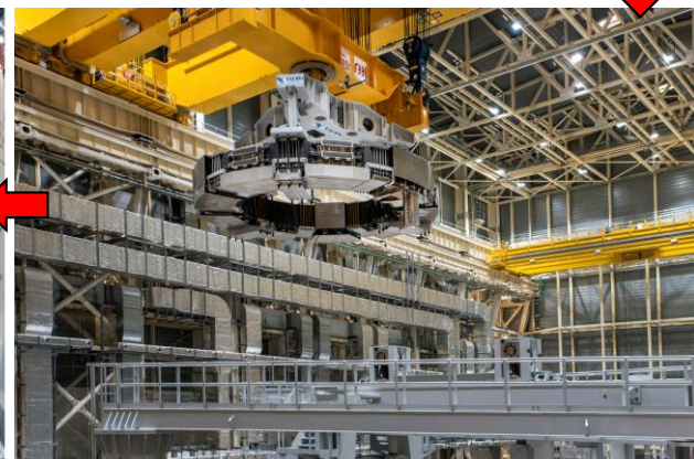
PF6 above Sector Sub-Assembly Tool
