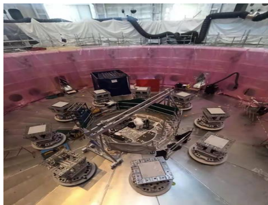
PF6 temporary supports in the PIT
