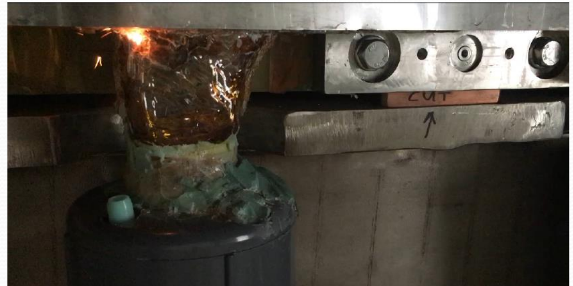
HiPot Test of CS Mock-Up: arcs between HV wires
