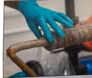
Technician applying insulation to an insulated break
